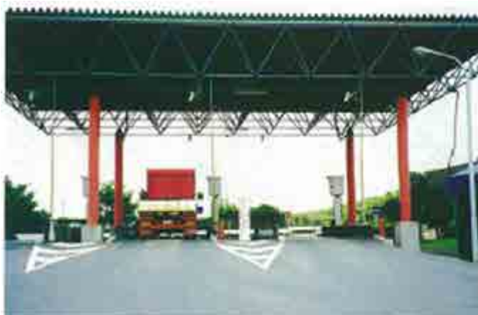
Weighing at the entrance gate
