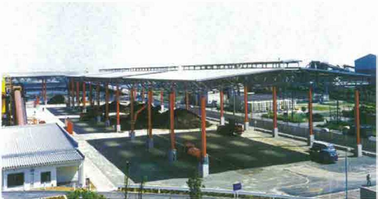
View of the entire yard for soil improvement
